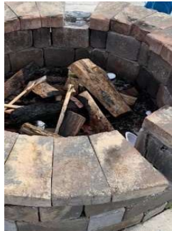
Loose and missing bricks on firepit
