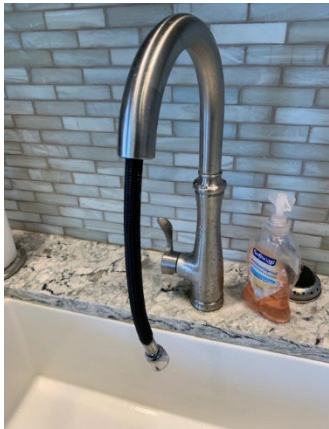
Broken spray hose in kitchen
