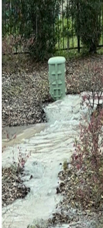
Irrigation main line break
