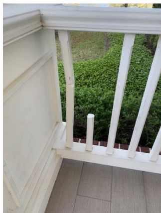
Railing at Manor House Porch needs repaired
