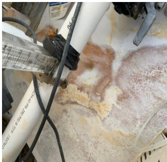
Leaking flow meter on pool equipment
