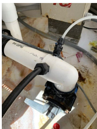
Replaced chlorine tubing on pool system complete
