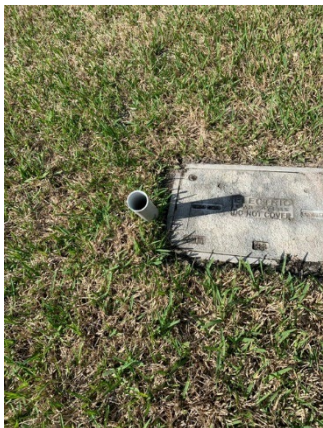
Electrical conduit left by contractor
