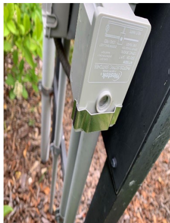
Replaced photo cell
