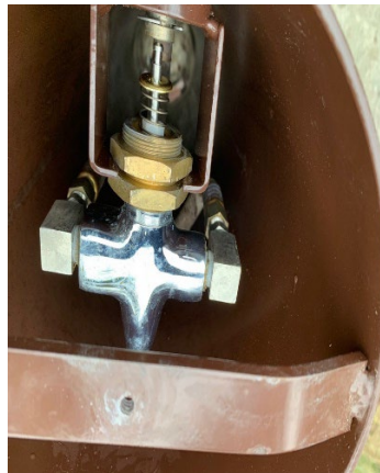
Replaced leaking valve
