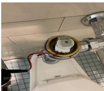
Repaired toilet flush valve
