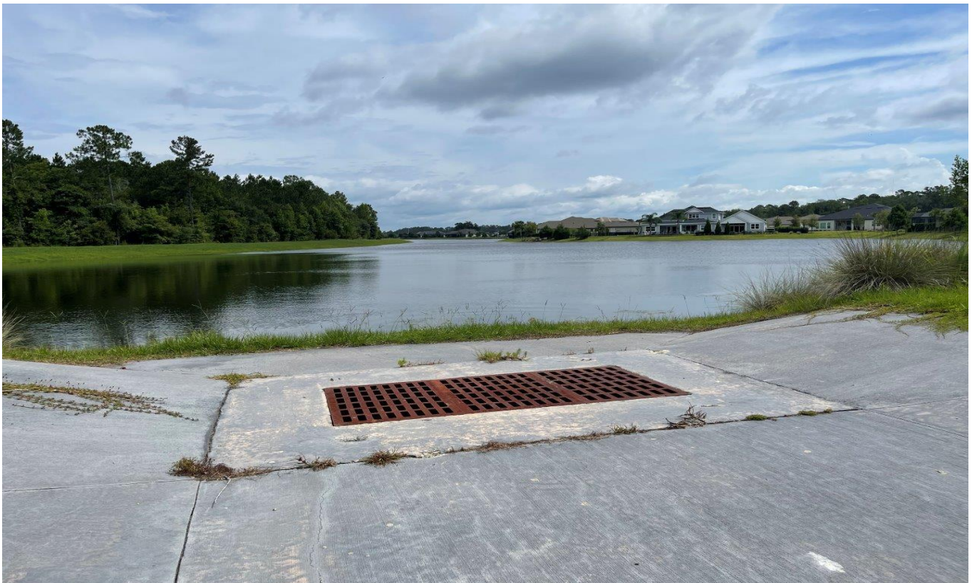
Storm Water Management Facility 2 Control Structure and Overflow Spillway (06-23-23)
