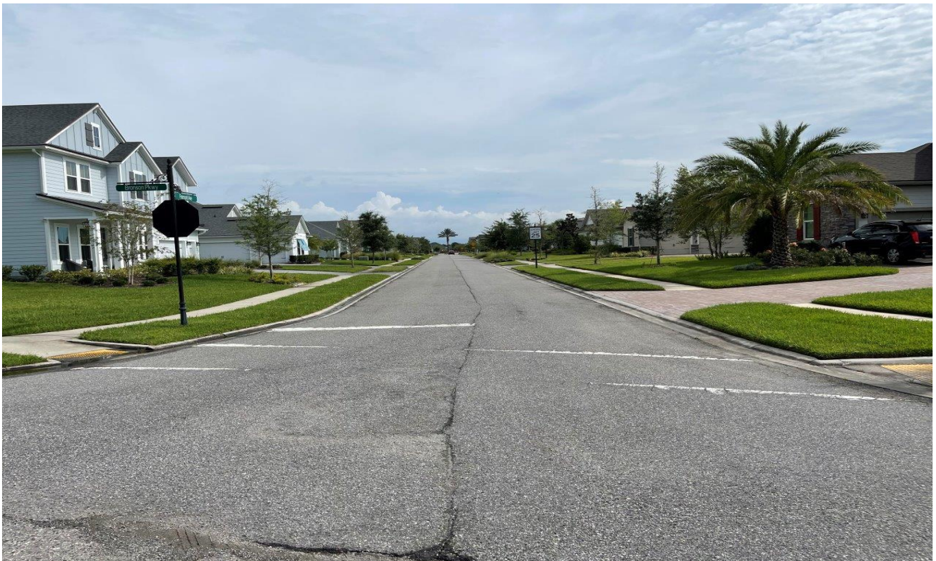
Fremont Avenue at Bronson Parkway (Striping fading and Repaired Potholes) (06-23-23)
