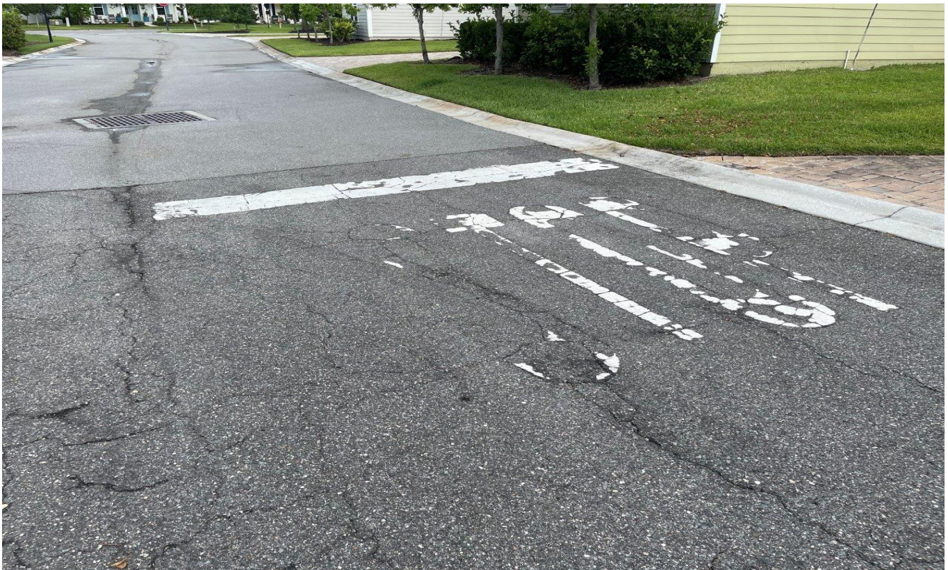
Roadway Striping fading on Roadways (06-23-23)
