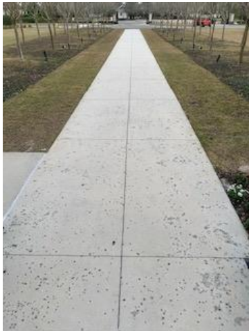
Finished pressure washing around the Manor house.
