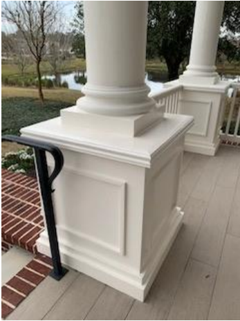
Cleaned and touched up the front columns.
